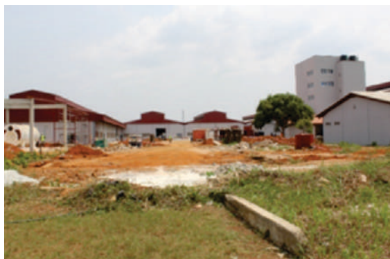
Outer view of the cashew Processing Factory
